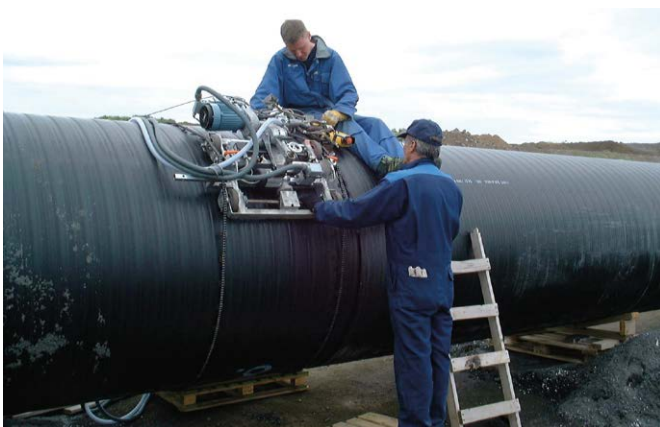
External welding machine
