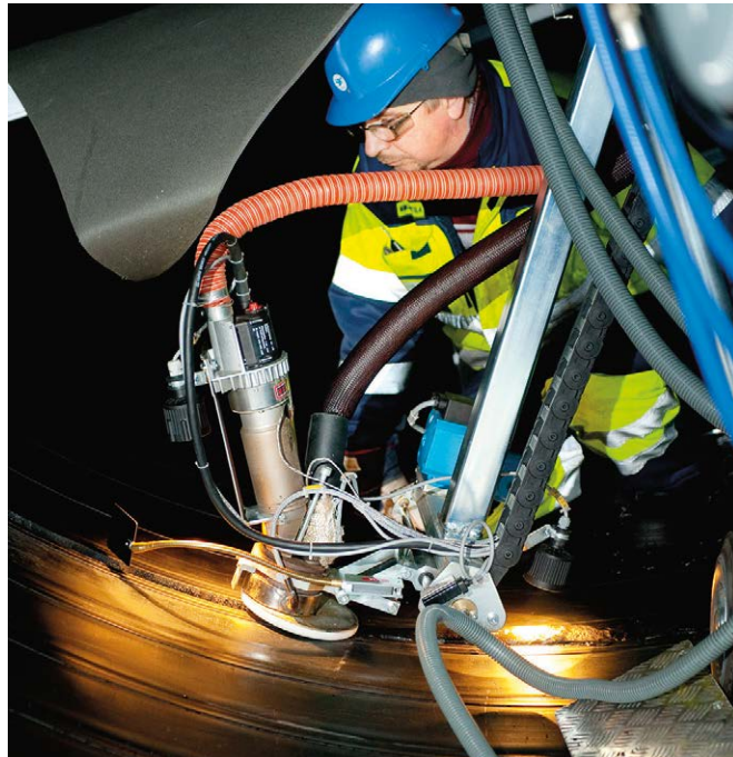
Internal extrusion welding machine. All works are to be carried out by experienced personnel.
