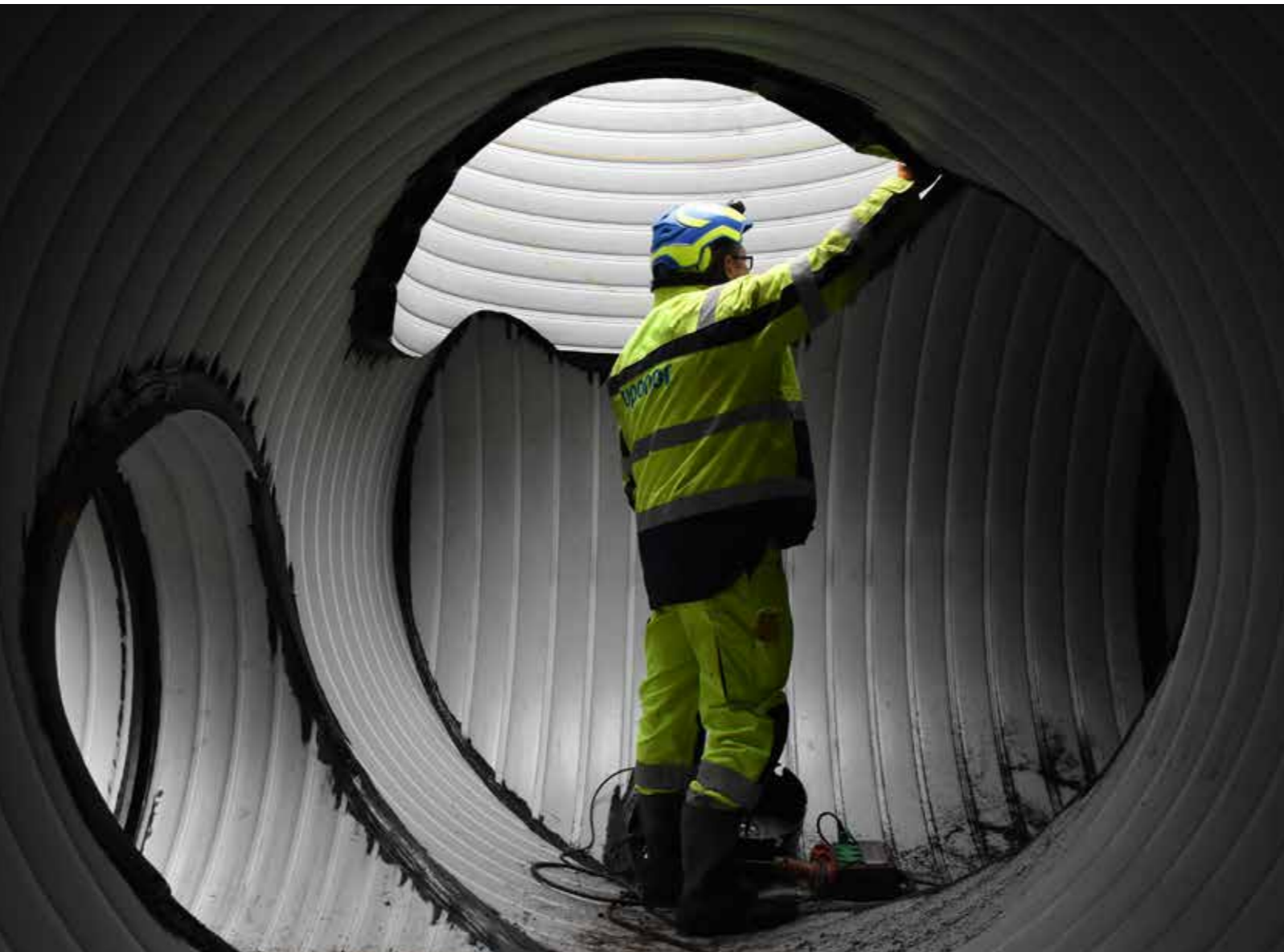
The long pipe lengths allowed Uponor's welders to assemble a complete tank quickly on site.
